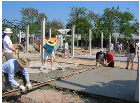
Starting to lay the slab on the first day
